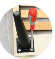
One screw on each side of the headboard are shorter  $(2 \times 5.5 cm)$  than the others on the sides of the bed  $(6 \times 6 cm)$
